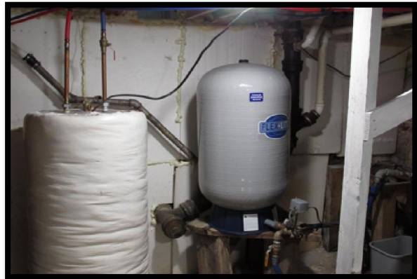
Water Heater and Well Pressure Tank in Basement
