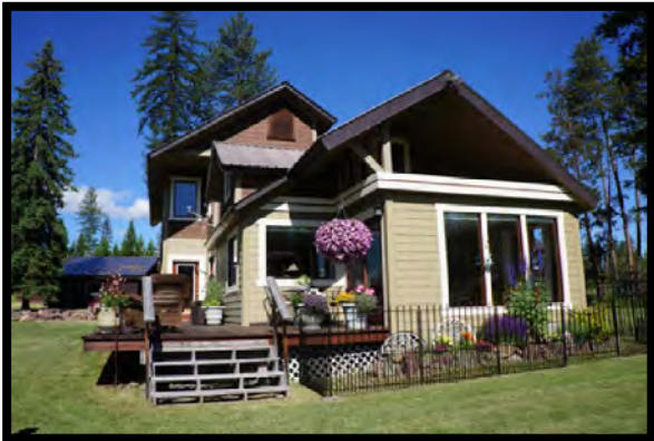
East Side of Residence
