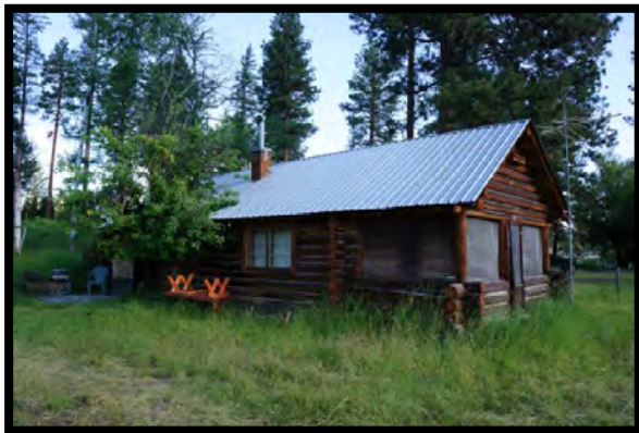
East and South Sides of Cabin
