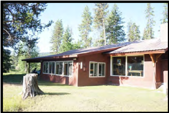
East Side of Residence
