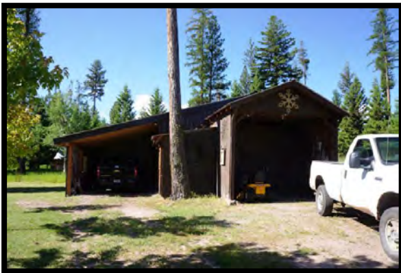
Garage/Storage Building Front
