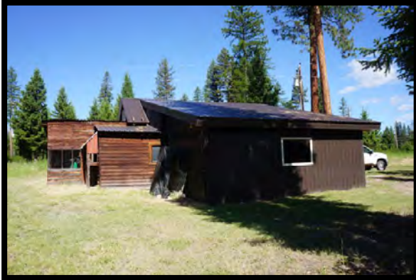
East Side of Garage/Storage Building
