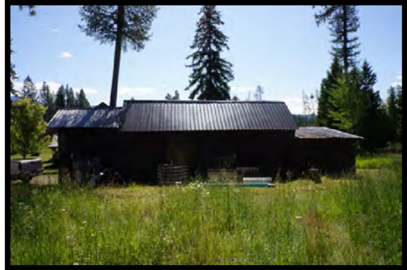
West Side of Garage/Storage Building
