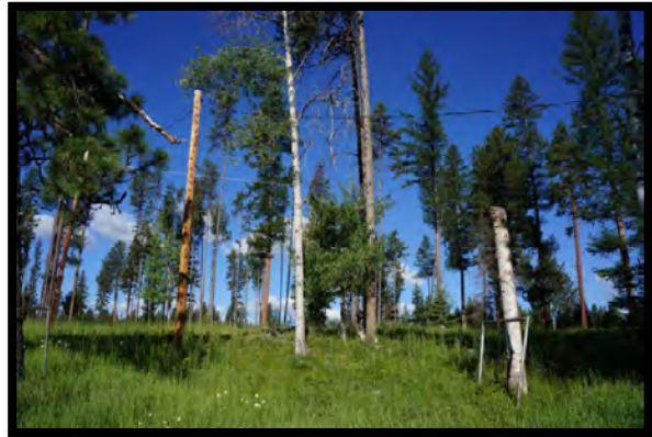
Power Transmission Lines on Lot 12
