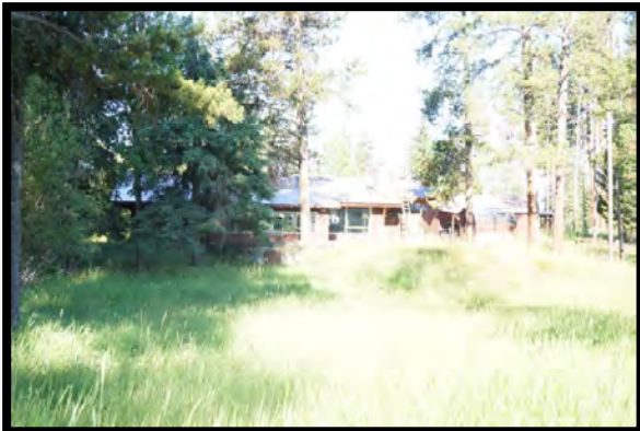
Residence on Lot 14 Looking West
