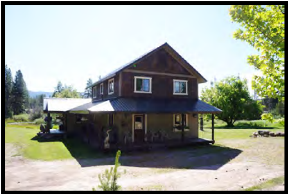
West Side of Residence
