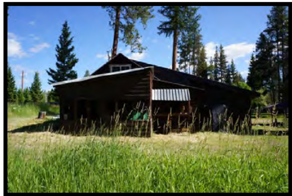
South Side of Garage/Storage Building
