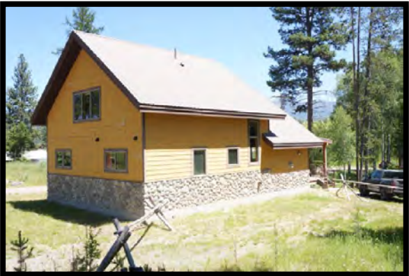
West and South Side of Residence
