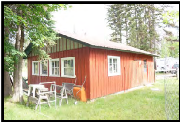
South and East Sides of Garage
