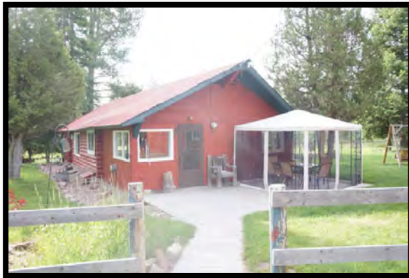
Entrance to Residence on Lot 15
