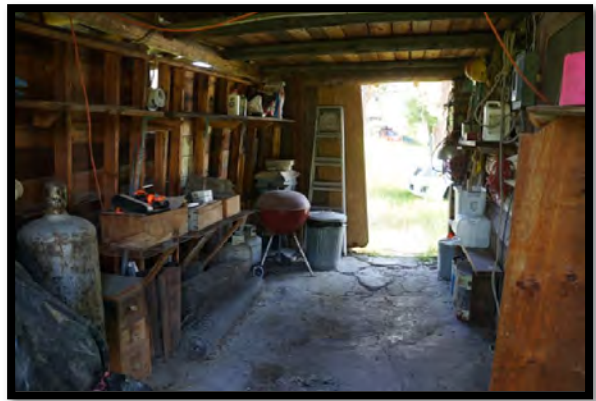
Enclosed Storage on West Side of Cabin
