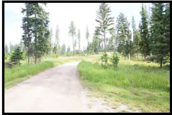
Cabin Site Access Road Looking North
