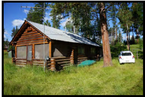
East and North Sides of Cabin
