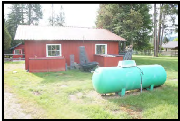
West Side of Garage
