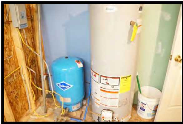
Water Heater and Pressure Tank
