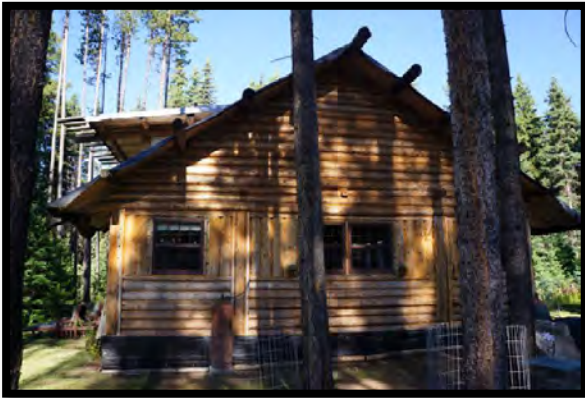
East Side of Residence
