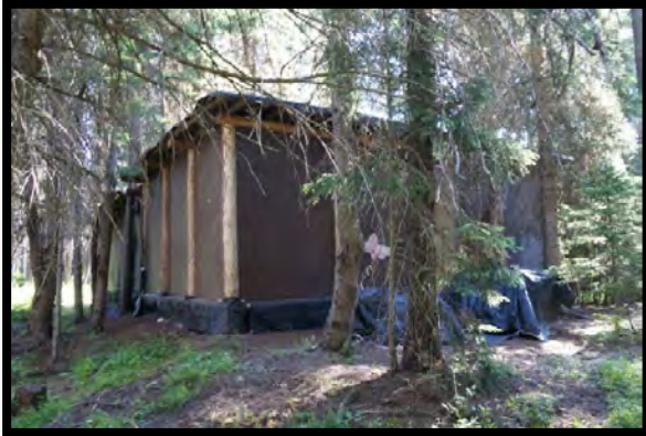
North Side of Storage Building
