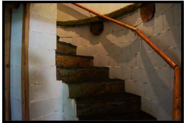
Stairs to Second Floor
