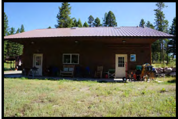
West Side of Detached Garage Building
