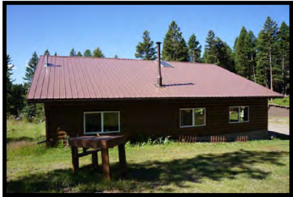
East Side of Garage/Apartment
