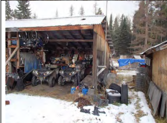
Open pole shed
