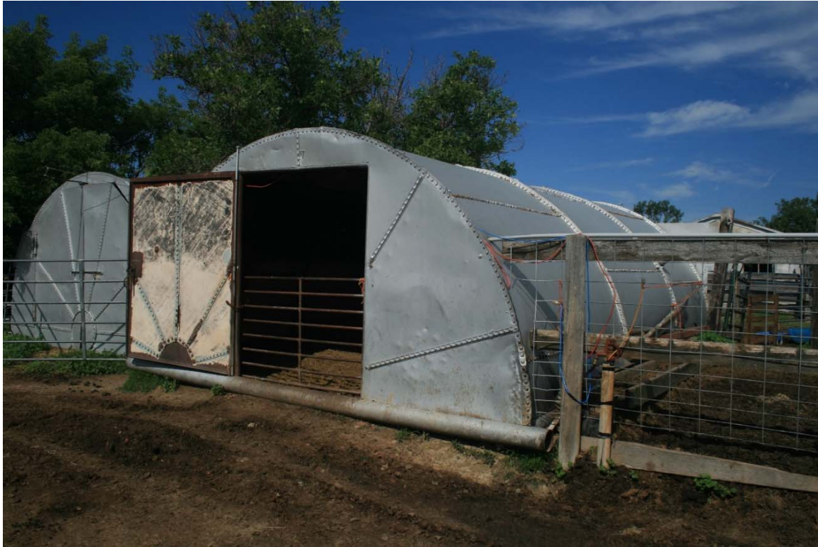
Oil tanks that have been cut in half and made into livestock sheds.
