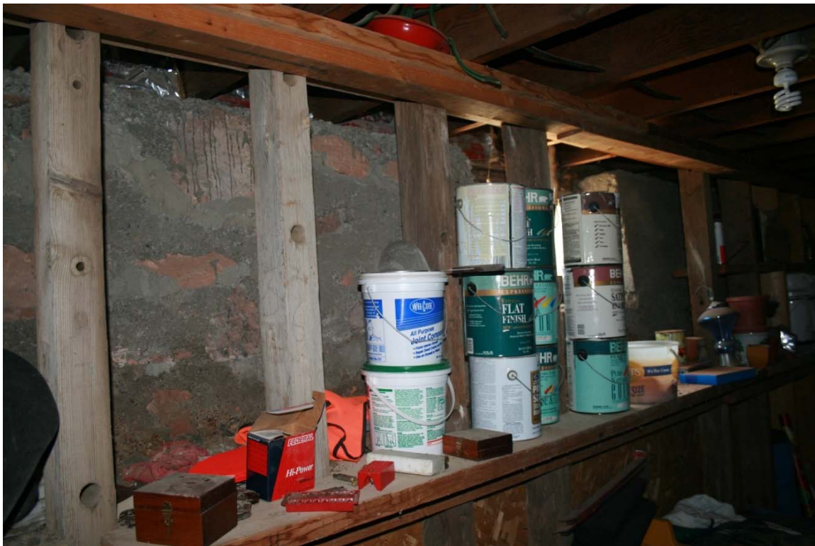
Foundation of the dwelling with supports added.
