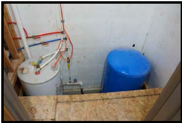
Water Heater and Pump Tank
