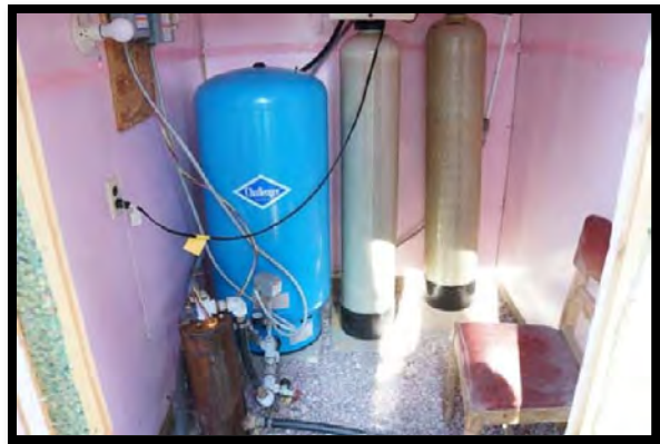
Water Pump and Softener Equipment
