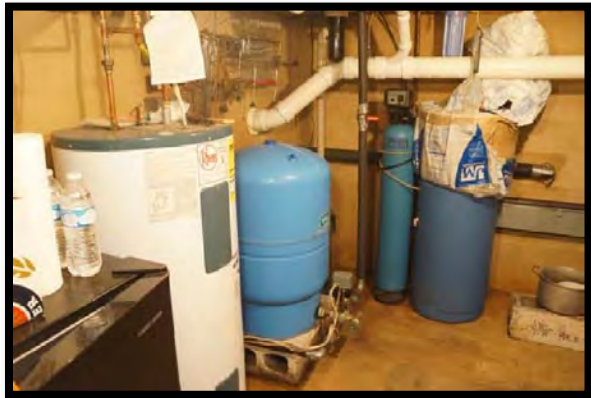
Water Heater and Softener
