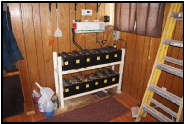
Batteries for Solar Power System
