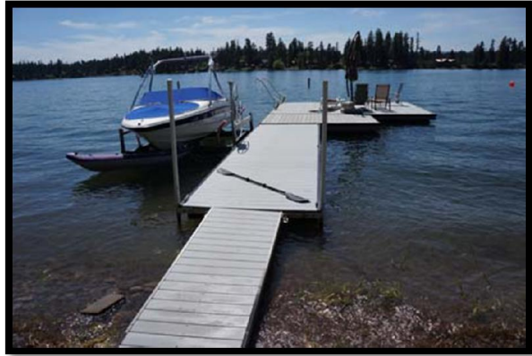
Pier and Floating Dock
