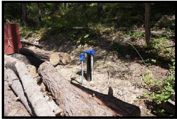
Newly Installed Well
