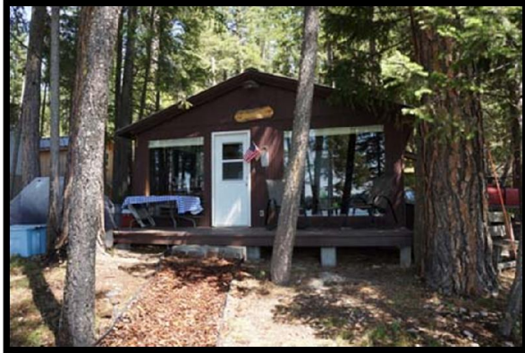
West Side of Residence on Lot 19
