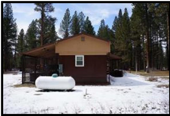
East Side of Residence
