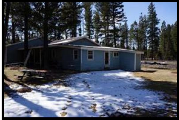
Rear of Residence Looking Southwest
