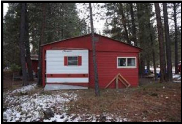
East Side of Residence
