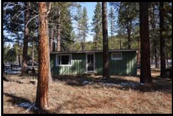
Front of Cabin on Lot 2 Looking North
