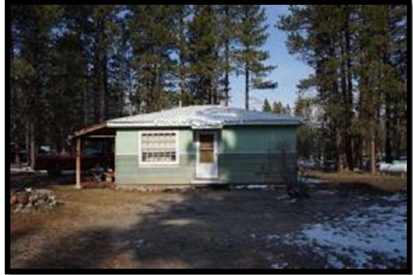
East Side of Residence
