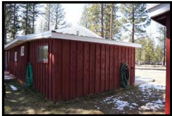
East Side of Residence
