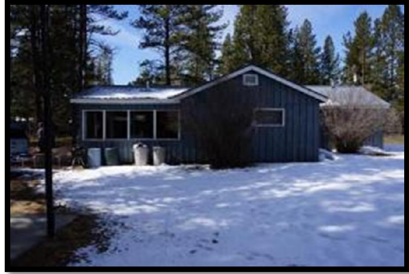
East Side of Residence
