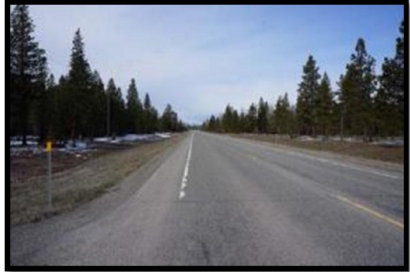
Montana Highway 200 Looking West
