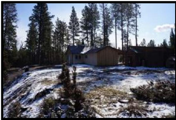
Lot 29 and Improvements Looking East
