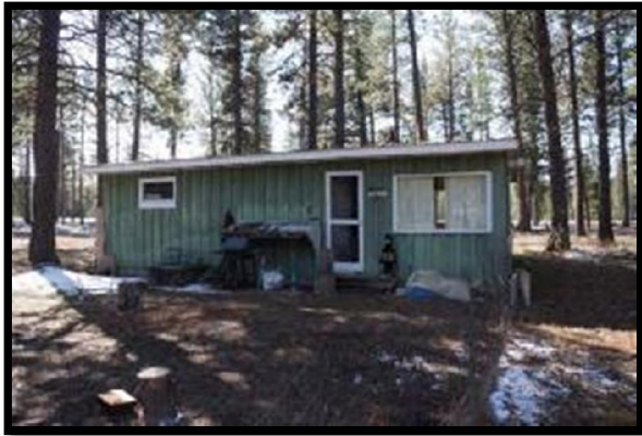
Rear of Cabin Looking South
