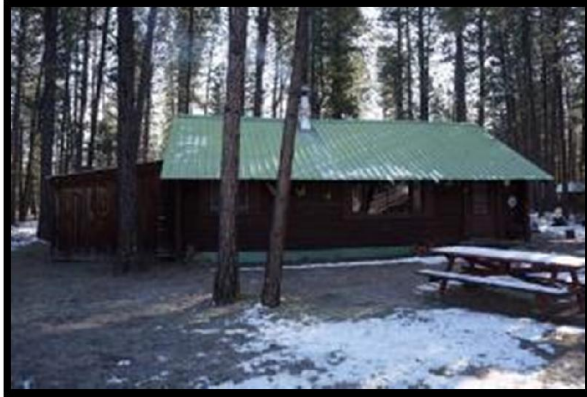
Front of Residence on Lot 9 Looking East
