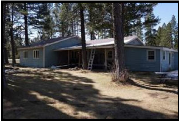
East Side of Residence
