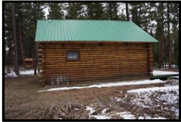
East Side of Residence
