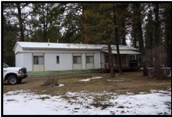
East Side of Residence
