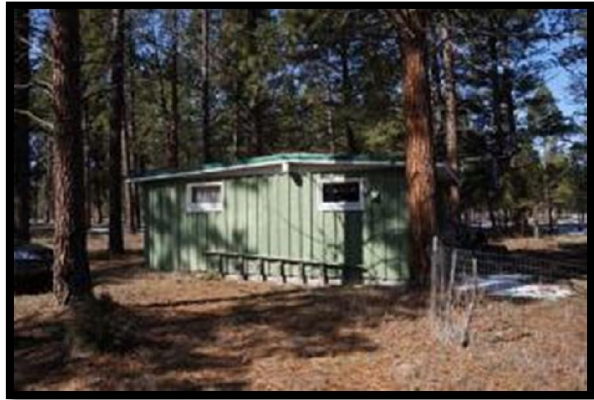
East Side of Cabin
