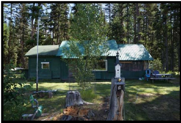
West Side of House
