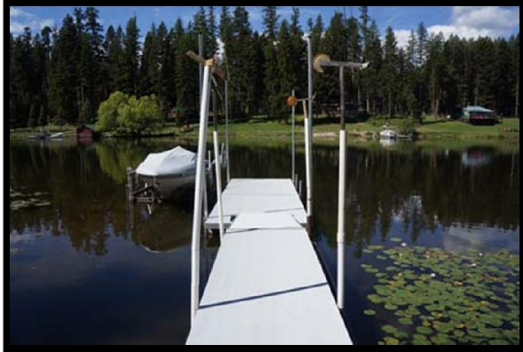
Pier and Dock
