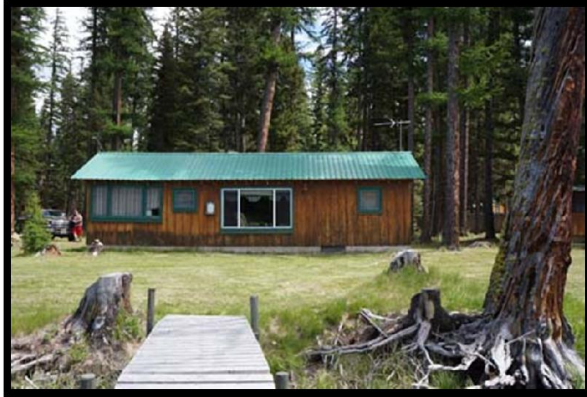
House on Lot 4 from Pier
