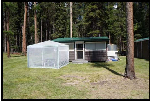
West Side of House on Lot 13
