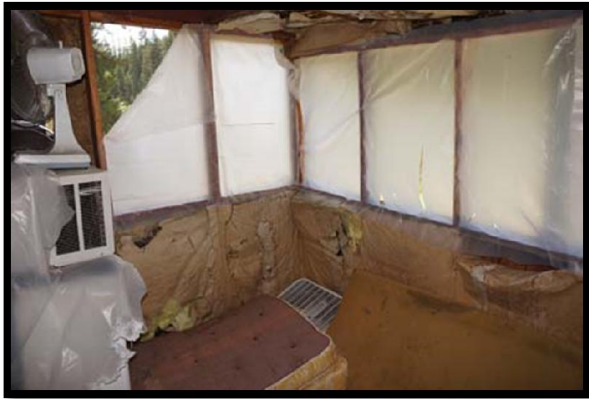
Bunk House 2 Porch
