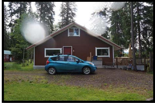
West Side of House
