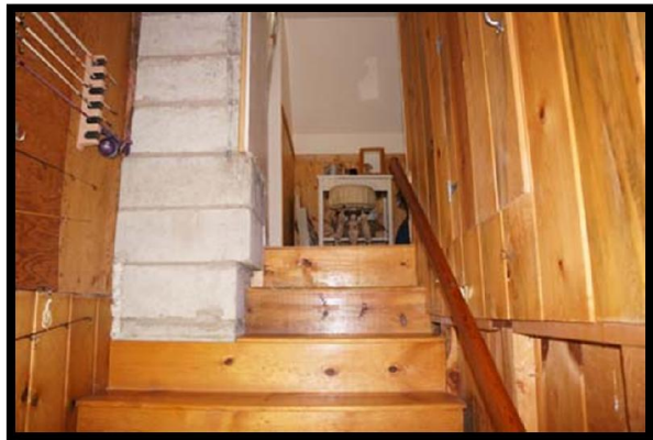
Stairs to 2 nd Floor
