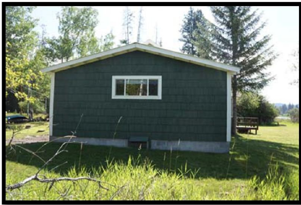
West Side of House
