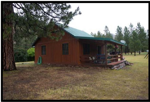
Side of Cabin and Covered Porch
