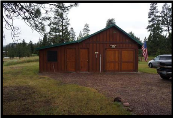
Front of Garage/Bunk House
