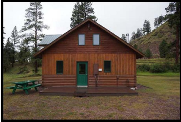
East Side of Cabin
