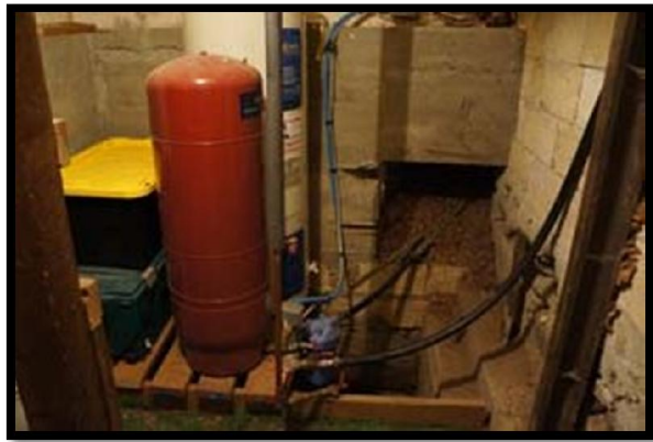
Water Heater in Crawlspace
