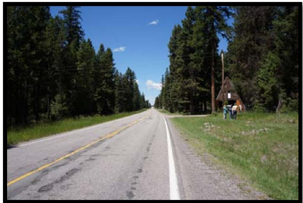
MT Highway 83 Looking North
