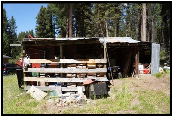
South Side of Shop/Storage Building
