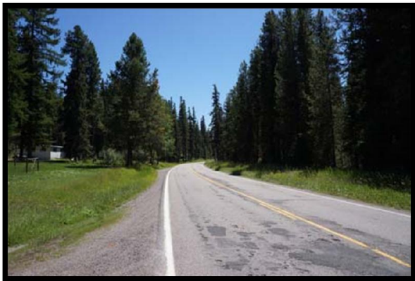
MT Highway 83 Looking South
