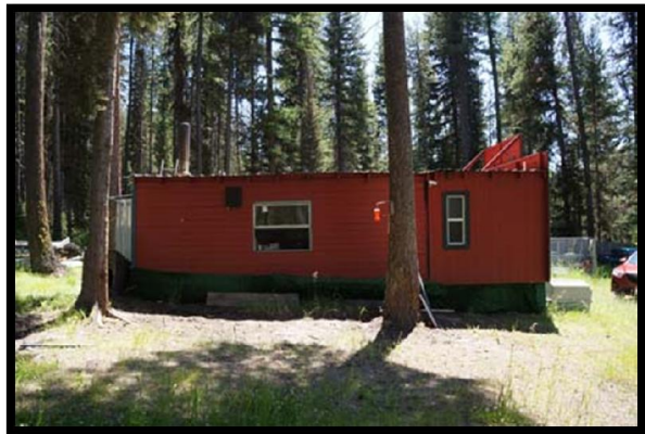
North Side of Shop/Storage Building
