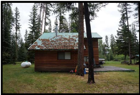
West Side of House
