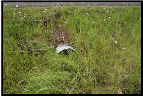
Drainage Culvert on North Portion of Property
