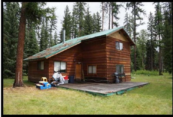
House and Deck
