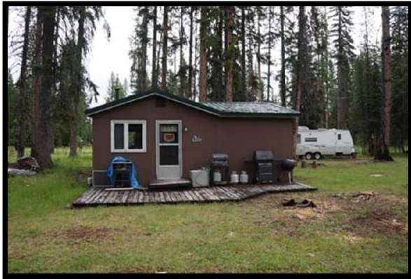
South Side of Cabin and Deck
