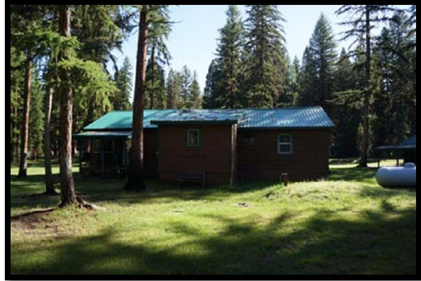
Rear of House
