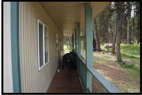
Covered Deck on North Side of House
