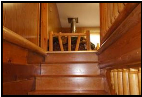
Stairs to Second Floor
