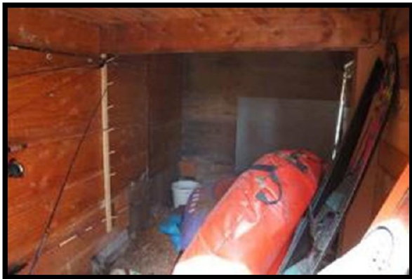
Storage Area under Screened Porch
