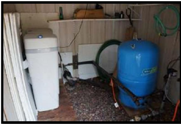
Pump House Interior
