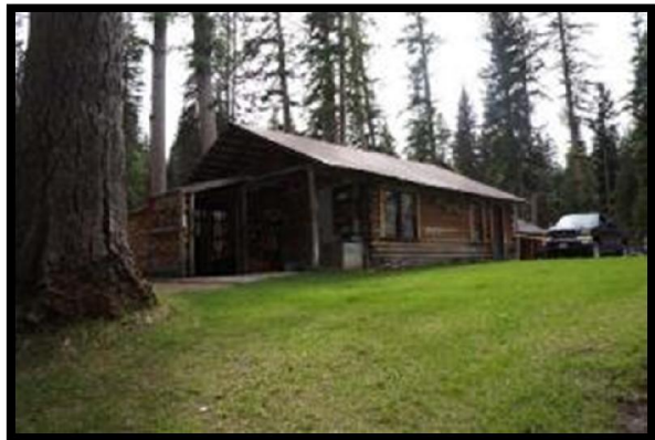
Former Forest Service Building/Garage
