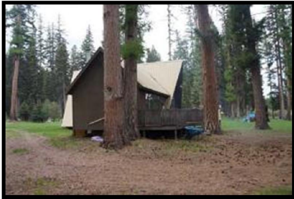
South Side of House
