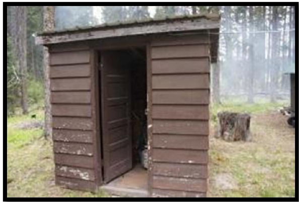
Former Pump House
