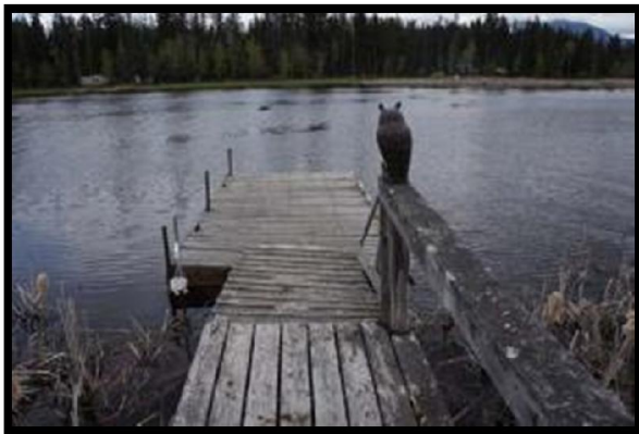
End of Pier and Floating Dock
