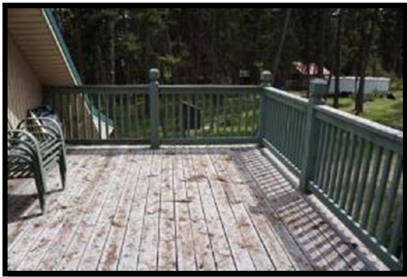
2 nd Floor Deck
