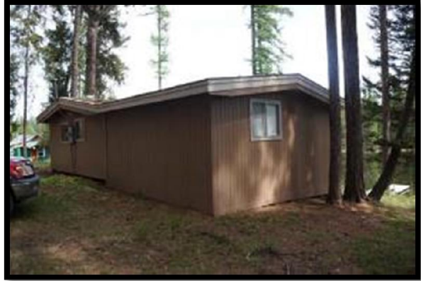
West and South Sides of Cabin
