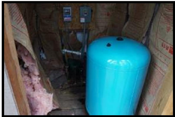
Pump House Interior
