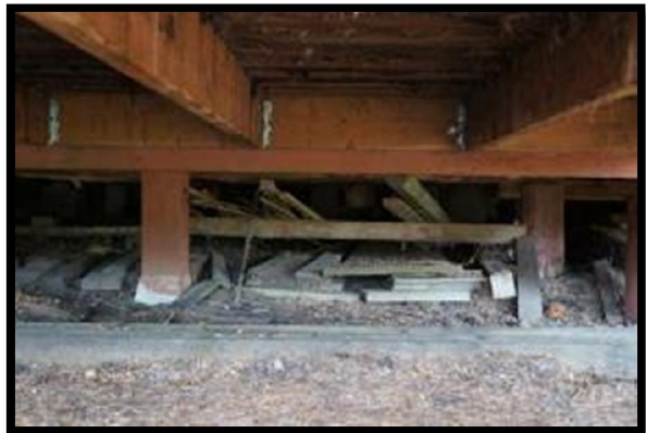
Post and Pier Foundation
