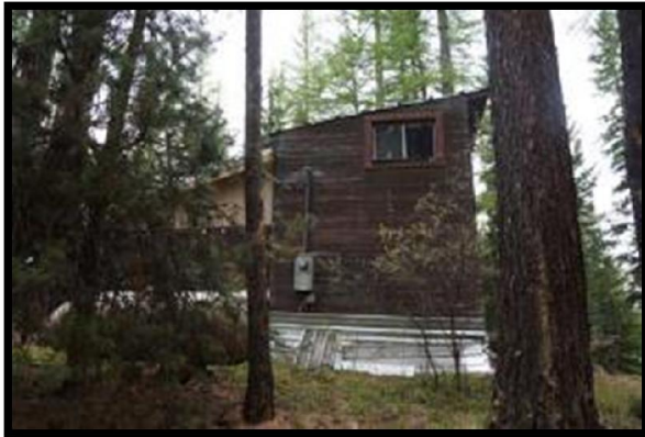
Southeast Side of Cabin
