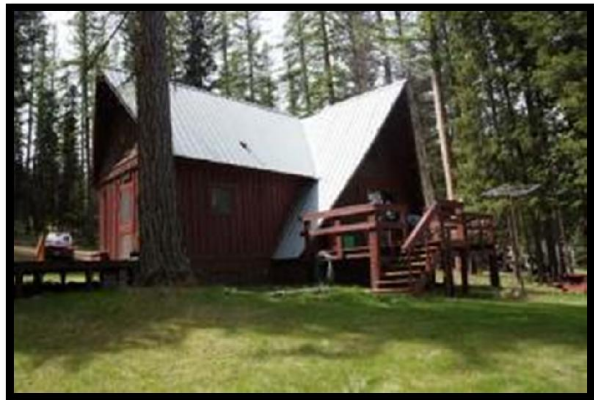
Front of Cabin Looking Southwest
