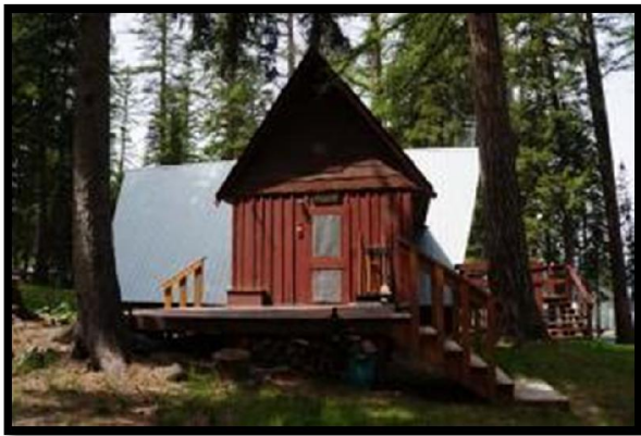
East Side of Cabin
