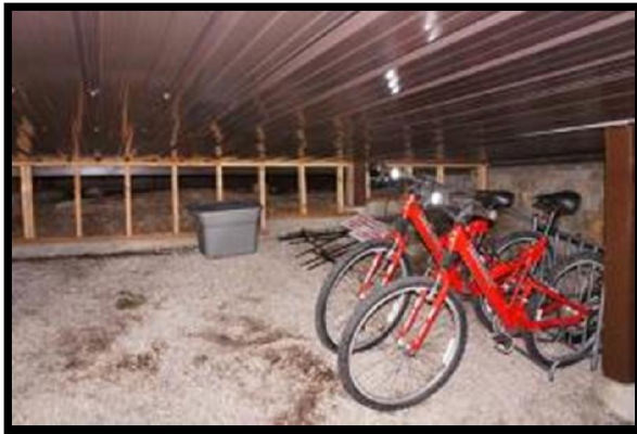
Storage Under Deck
