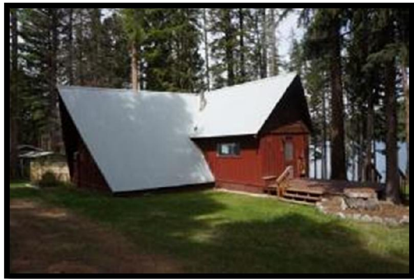
South and East Sides of Cabin
