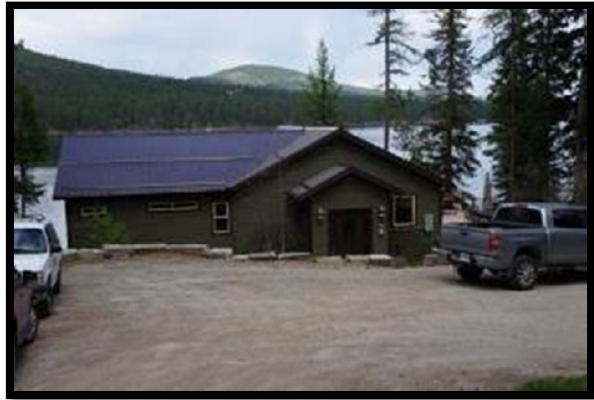
Rear of House and Parking Area
