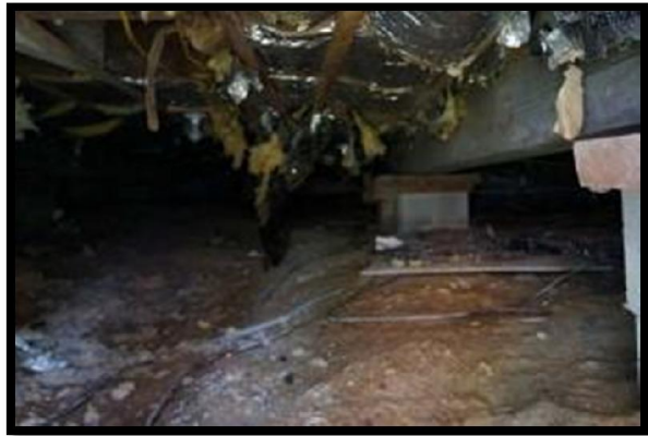
Cabin Pier Foundation
