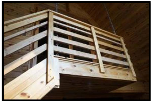
Stairs to Upper Level
