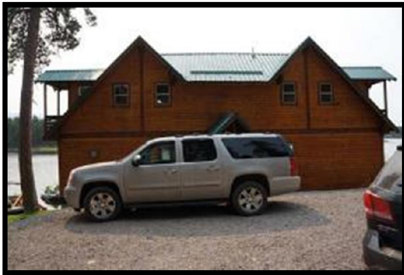
North Side of House and Parking Area
