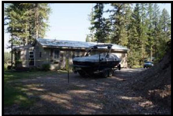
Rear of House and Gravel Parking Area
