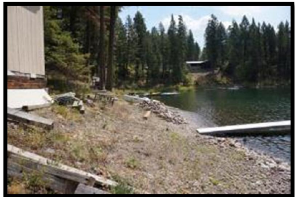
Lake Frontage Looking South
