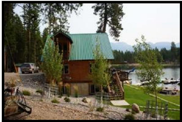
West Side of House and Landscaping
