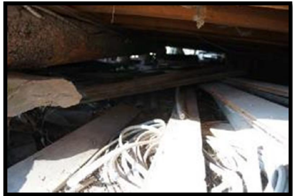
View of Foundation
