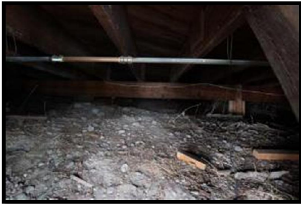
Cabin Pier Foundation
