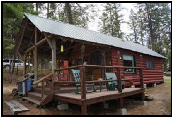
Deck and West Side of Cabin
