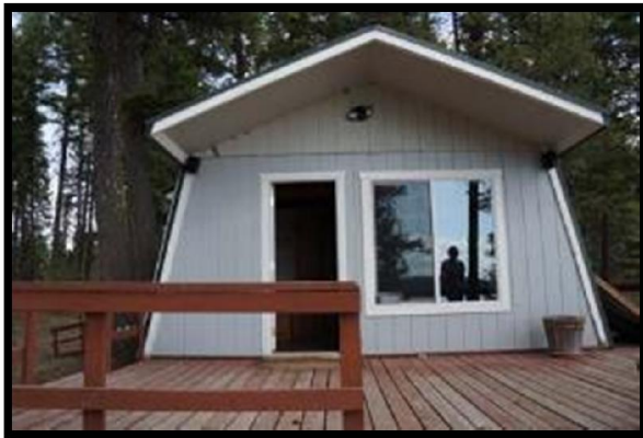
South Side of Cabin and Deck
