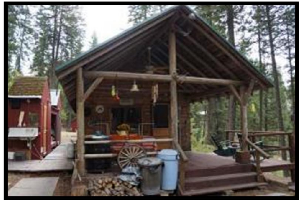
Front of Cabin and Deck
