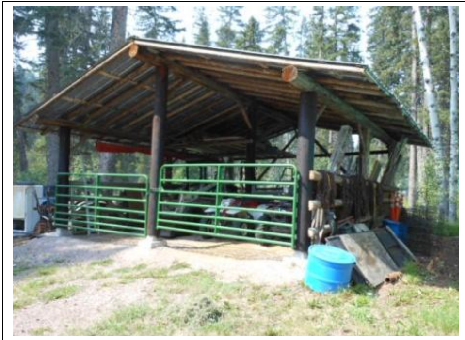
Subject pole building with gravel floor
