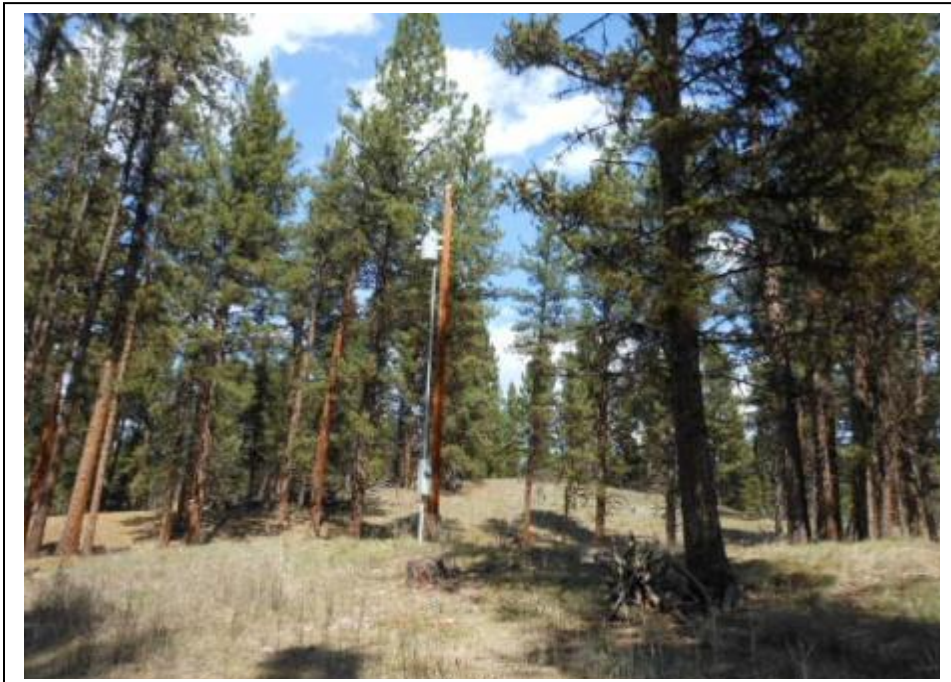
Subject power pole with underground power trenched to the cabin
